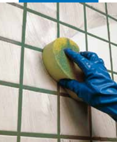
Cleaning and finishing the tile joints on a wall with a sponge
