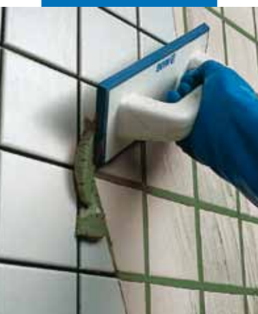
Spreading Ultracolor Plus on a wall with a rubber float
