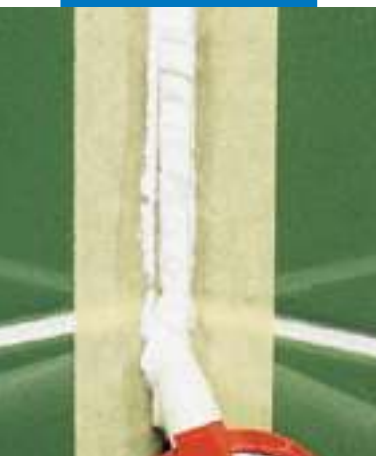
Application of Mapesil AC
