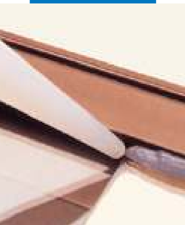
Sealing aluminium window frame with Mapesil AC
