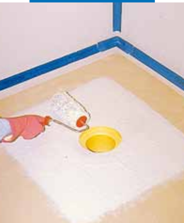
Spreading Mapegum WPS around the drain in a shower cubicle
