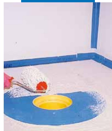
The special piece of Mapeband embedded in the Mapegum WPS
