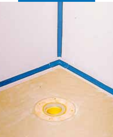
Bathroom wall waterproofed with Mapegum WPS and Mapeband
