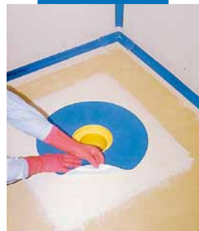
Positioning the special piece of Mapeband over Mapegum WPS
