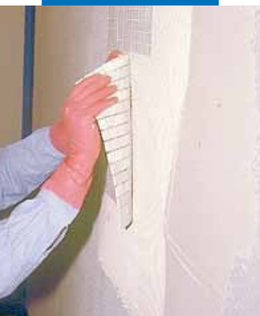
Laying glass mosaic
